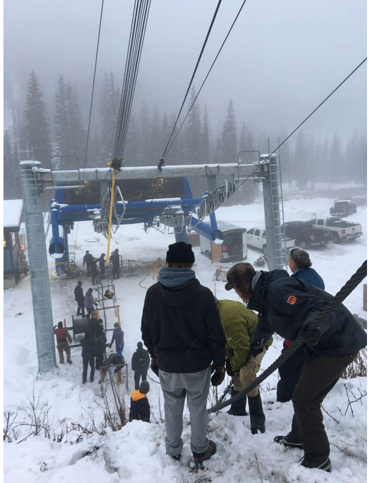
SROAM class assisting with the cable splice of the new Whitewater Raven chair, November 2023
